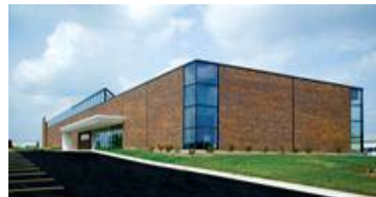
Reagent production plant in Chicago
