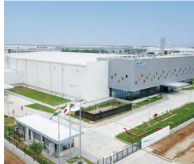
Establishment of a new production base in India in preparation for future growth
