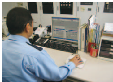
Introduction of electric power monitor at Technopark to determine status of electricity use throughout the facility
